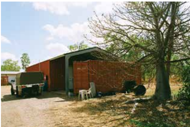
Nigel built his jerky manufacturing facility at Humpty Doo, 40km south of Darwin.
